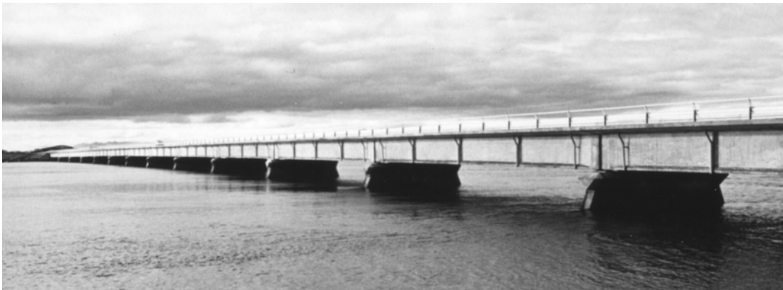
Figure 1. The 520 m long bridge on the Icelandic highway, 50 km from Reykjavik.
