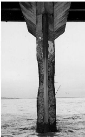
Figure 2. Front view of the deteriorated pillars.
