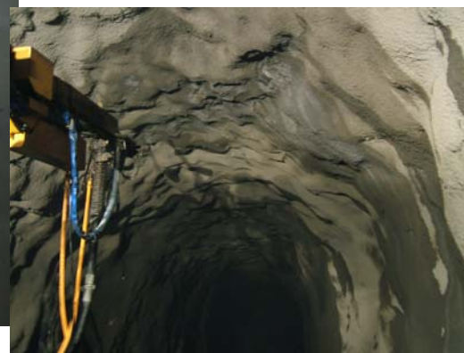
6-3-2006 During shotcreting w. 1 % XYPEX
