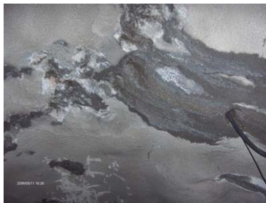
11-5-2006 2 months after shotcreting
